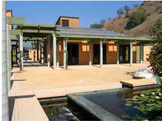
(c) EHDD Architecture/Solterra, LLC
