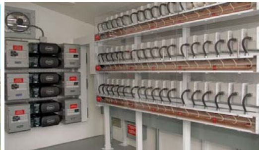
Photo: Anaheim Energy Park 75 kW PV panel with 54 kW hours of lithium ion battery storage backup
